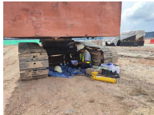
PLATE BEARING TEST
