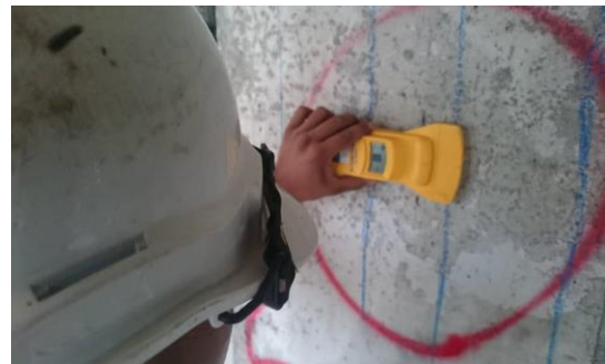
COVER METTER TO SCAN STEEL BAR POSITION
